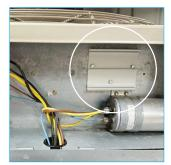
Install mounting bracket. Bracket can be mounted vertically or horizontally
