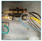
Remove compressor Run Wire (yellow in this example) from the contactor or terminal, as applicable
