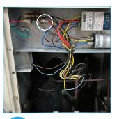
Red wire from AirGo active to loadside contactor, labeled 23 in this application
