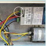
Strip the compressor Run Wire at least 1/2". Terminate wire in Run Winding terminal on AirGo
