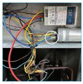
Terminate blue wire from AirGo to "H" on the capacitor
