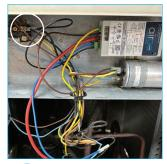
Black wire from AirGo to loadside contactor labeled 21 in this application
