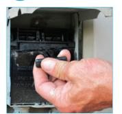
Turn off power to the HVAC unit at the circuit breaker or disconnect
