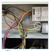
Terminate brown wire from AirGo to "C" on the capacitor
